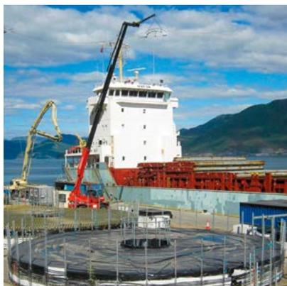
The Jayabaya cable on Java Island will provide high-speed Internet between Jakarta and Surabaya via Cirebon and Semarang. Nexans supplied PT Mora Telematica Indonesia with 950 km of 24-core unrepeated (URC-1) fiber-optic cable. Installation was scheduled for completion in November 2018.
