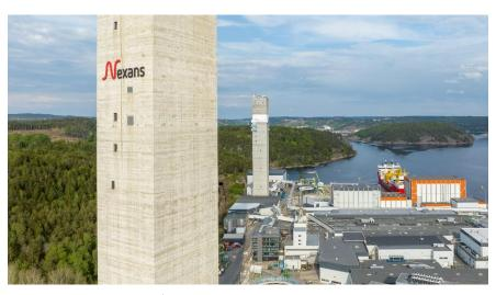
second extrusion tower which will allow the plant to insulate four cables simultaneously in addition to the two existing lines and qualifies as Norway's tallest building and first skyscraper.
